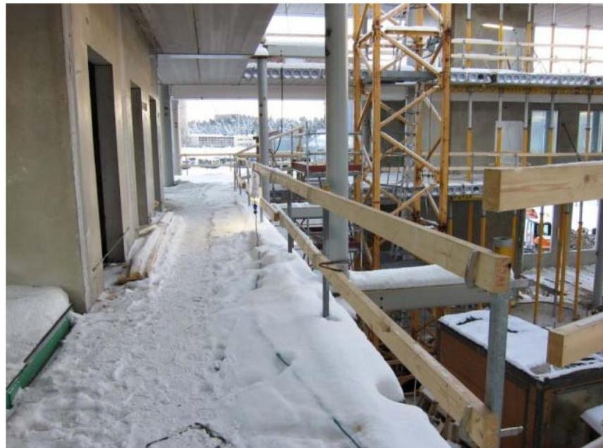
Figure 48. Comparing model and live situation: The final handrails of the building were intended to be used as falling prevention in construction phase.
